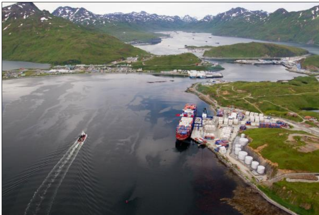
Figure 2. View of a container ship berthed at the CMA CGM Dutch Harbor Terminal (Photo credit: Dan Parrett, City of Unalaska).
