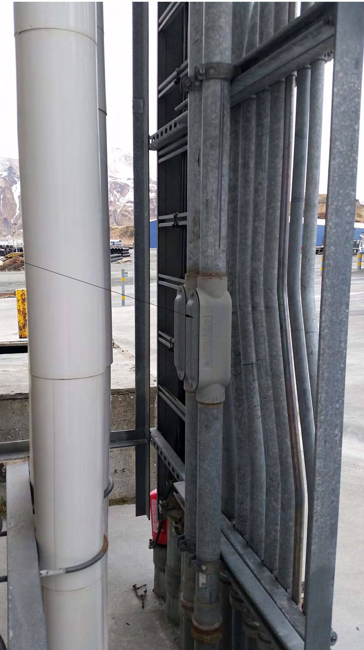
PICTURE 2: OLD POWERHOUSE SPARE CONDUITS
