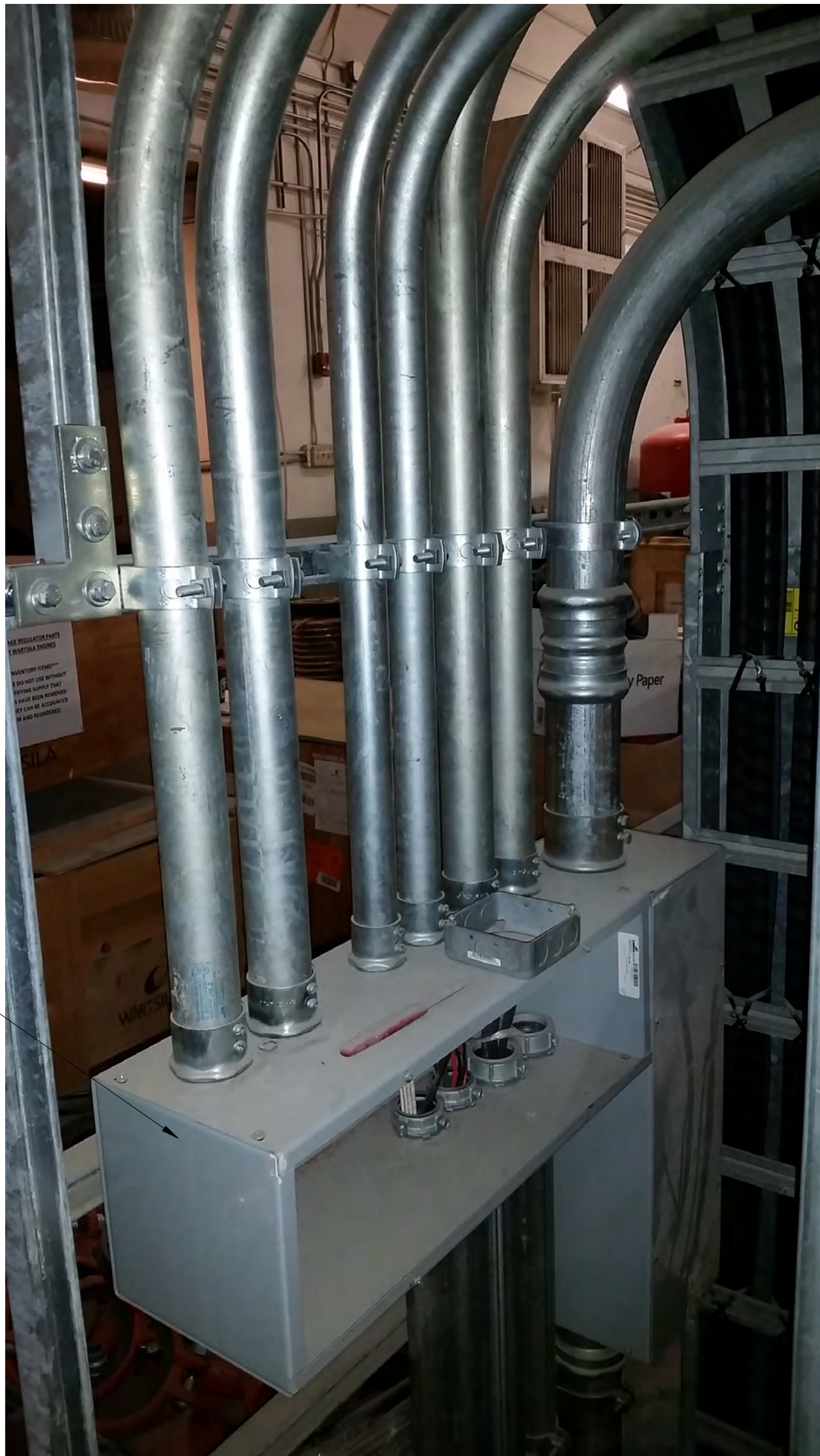
PICTURE 3: OLD POWERHOUSE SECOND FLOOR
