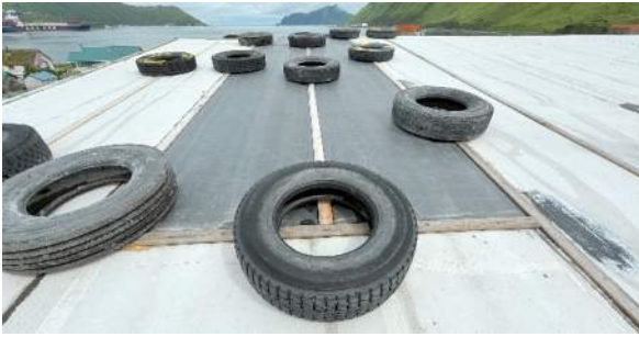
Photo #31: Area of Repair Weighted Down with Tires and Battens Surface Fastened
