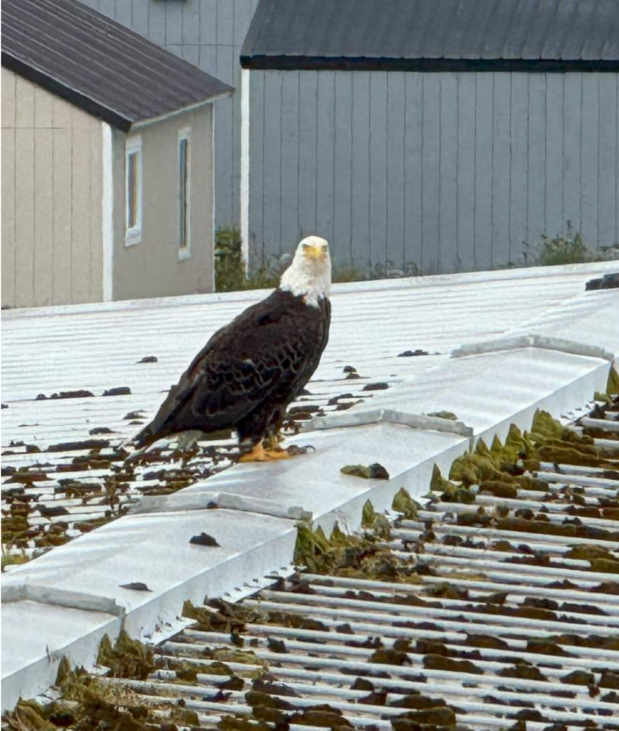
Photo: Site visit was accompanied by drop-in roof consultant.
