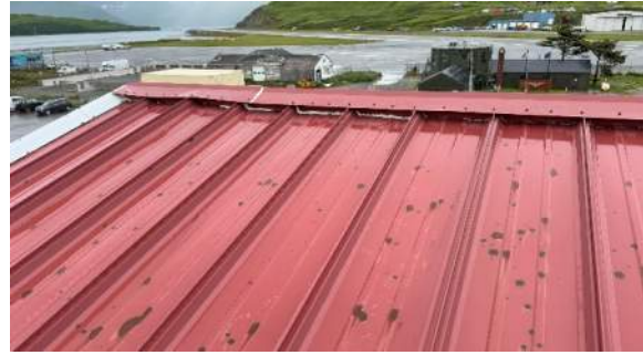
Photo #4: Metal closure panel at ridge re-sealed
