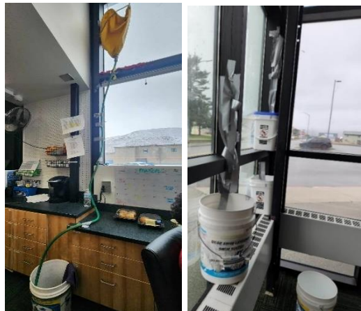
Figure 9: Leaks in offices and lobby
