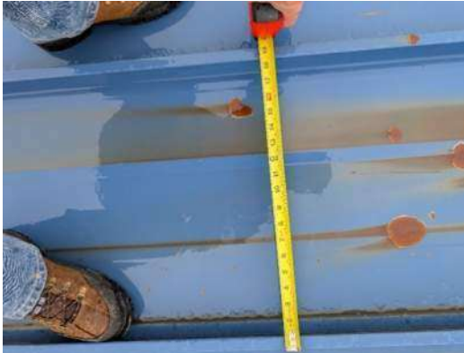
Photo #1: Corrosion on metal roof
