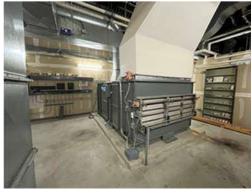
Photo #6: Typical AHU
