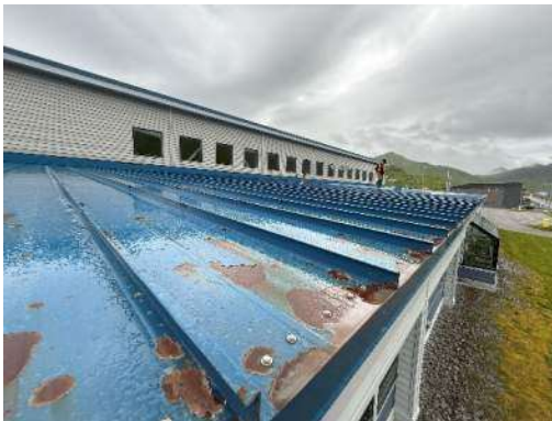
Photo #3: Corrosion on metal roof
