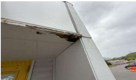
Photo #5: Degraded soffit
