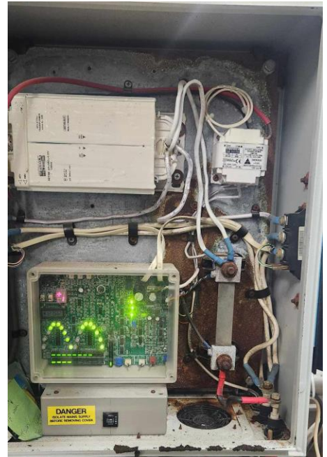
Figure 11: Corroded Pump Room equipment.
