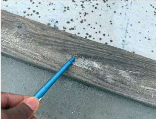
Photo #1: Corroded fastener
