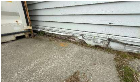
Photo #9: Exposed insulation at wall
