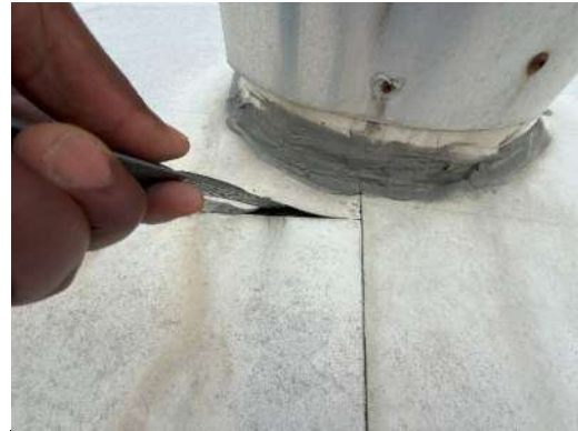
Photo #2: Failed seam
