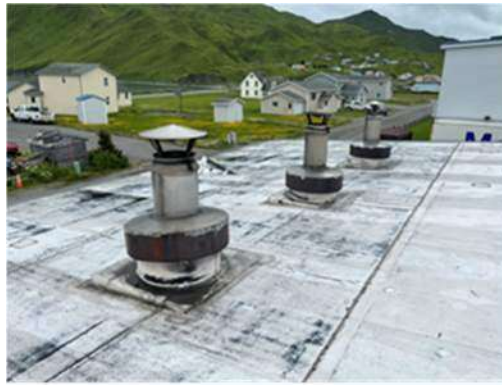
Photo #2: Exterior boiler flue
