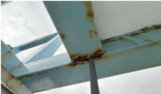
Photo #17: Corroded structure
