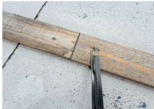
Photo #8: Loose fasteners
