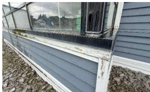
Photo #10: Degraded trim at wall
