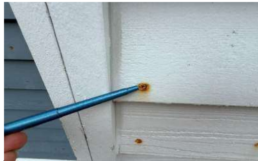
Photo #12: Corroded fasteners at wall
