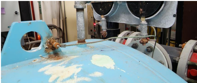
Photo 4b (Example of incorrect wire used for bonding. Should be solid not stranded)
