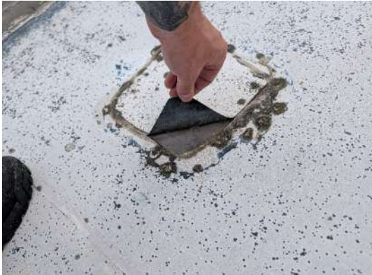
Photo #5: Failed repair
