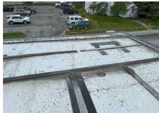
Photo #4: Degrading membrane seams
