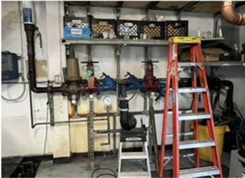
Photo #9: Domestic cold water header
