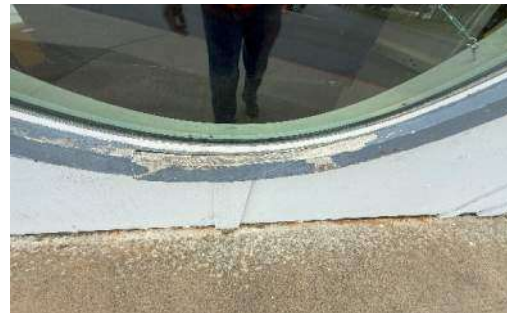
Photo #6: Degraded paint
