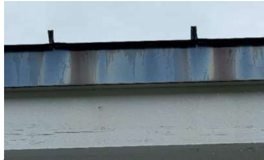
Photo #18: Corroded fascia
