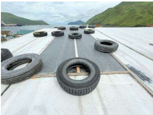
Photo #7: Unadhered membrane on roof
