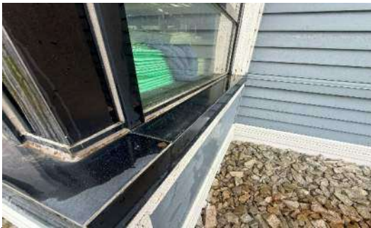
Photo #15: Corroded fasteners at sill
