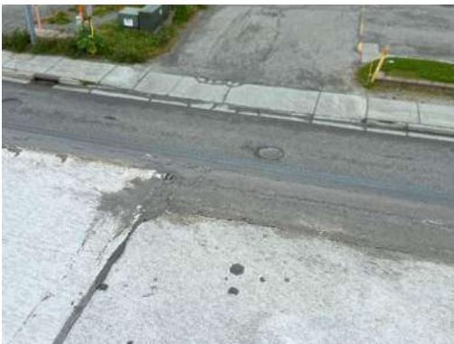
Photo #3: Degrading membrane
