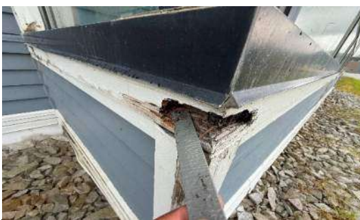
Photo #11: Degraded trim at wall
