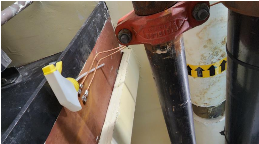
Photo 4a (Example of bonding wire terminated incorrectly)
