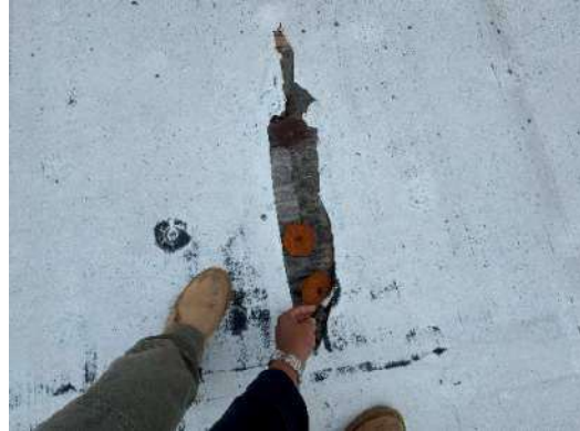
Photo #6: Exposed substrate
