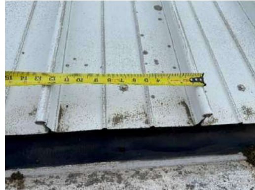
Photo #2: Corrosion on metal roof
