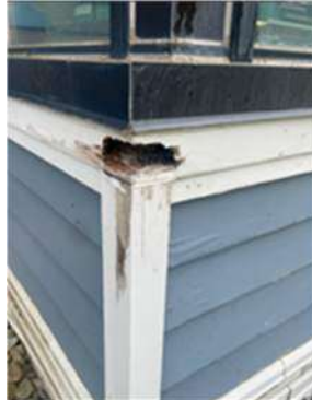
Photo #2: Degraded sill
