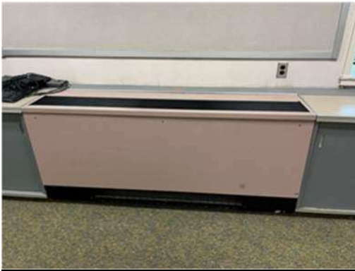
Photo #3: Typical classroom unit ventilator
