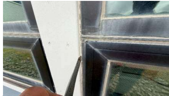
Photo #16: Failed sealant joint
