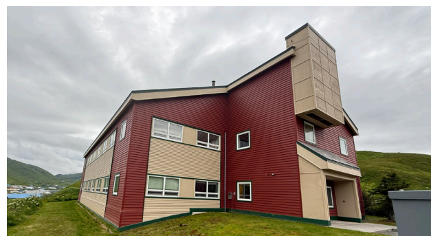
Unalaska City Hall Roof Assessment 2025 (Unalaska, AK)
